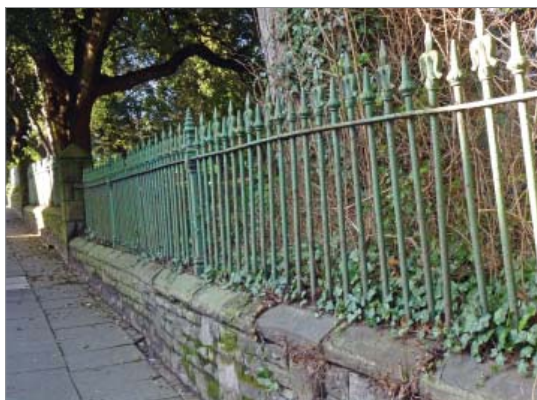
The listed railings around St James's Churchyard
