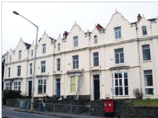
Nos. 94-96 consec Walter Road and No. 43 St James Crescent
